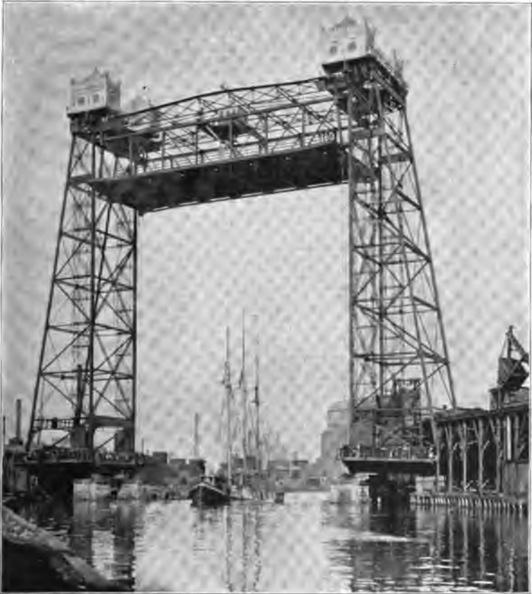
PLATE I. TRANS. AM. SOC. CIV. ENGRS. VOL. XXXIII, No. 742. WADDELL ON HALSTED STREET LIFT-BRIDGE.
